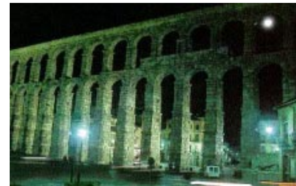
Segovia, the Roman Aqueduct
